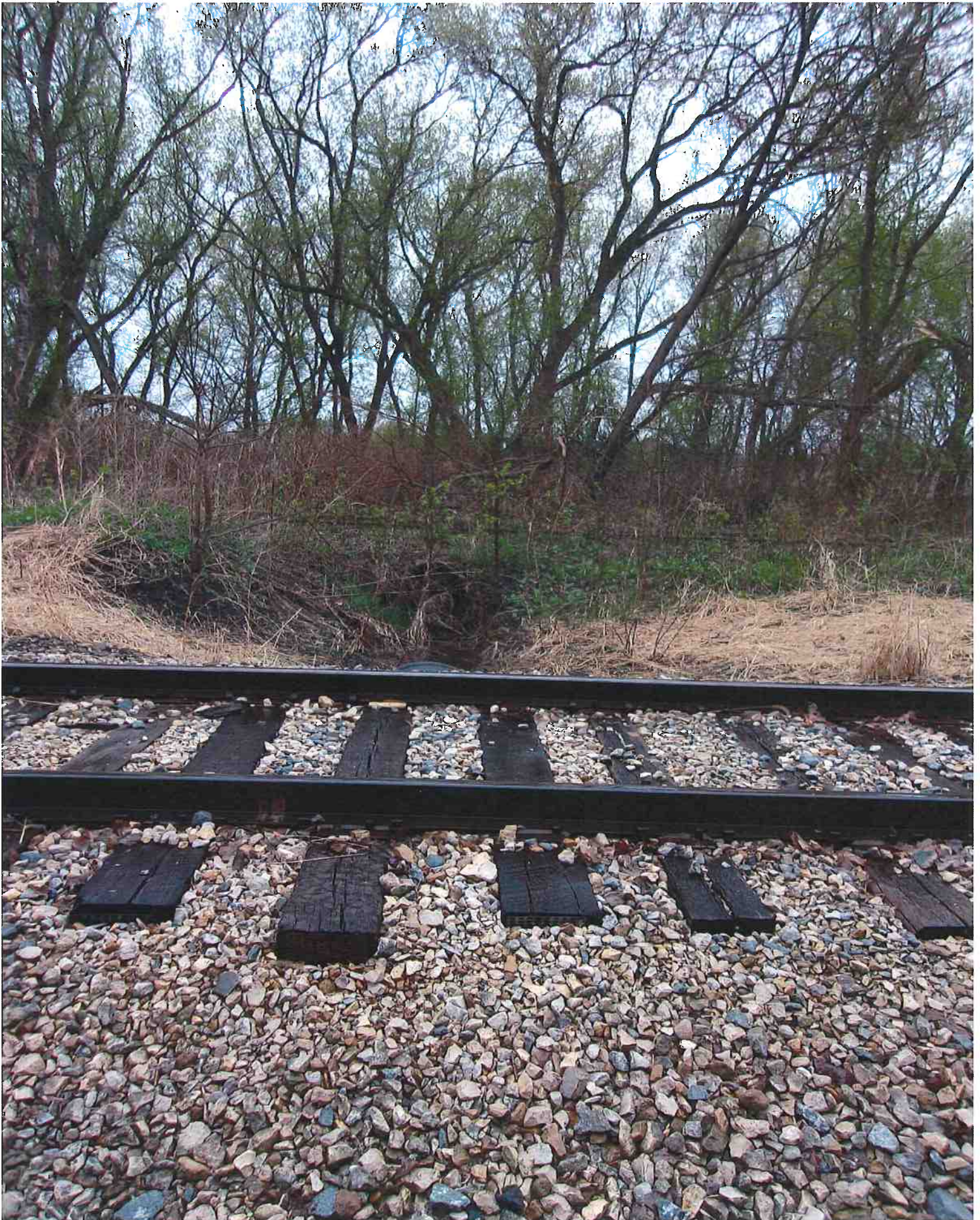
Looking upstream towards Georgetown Rd.
