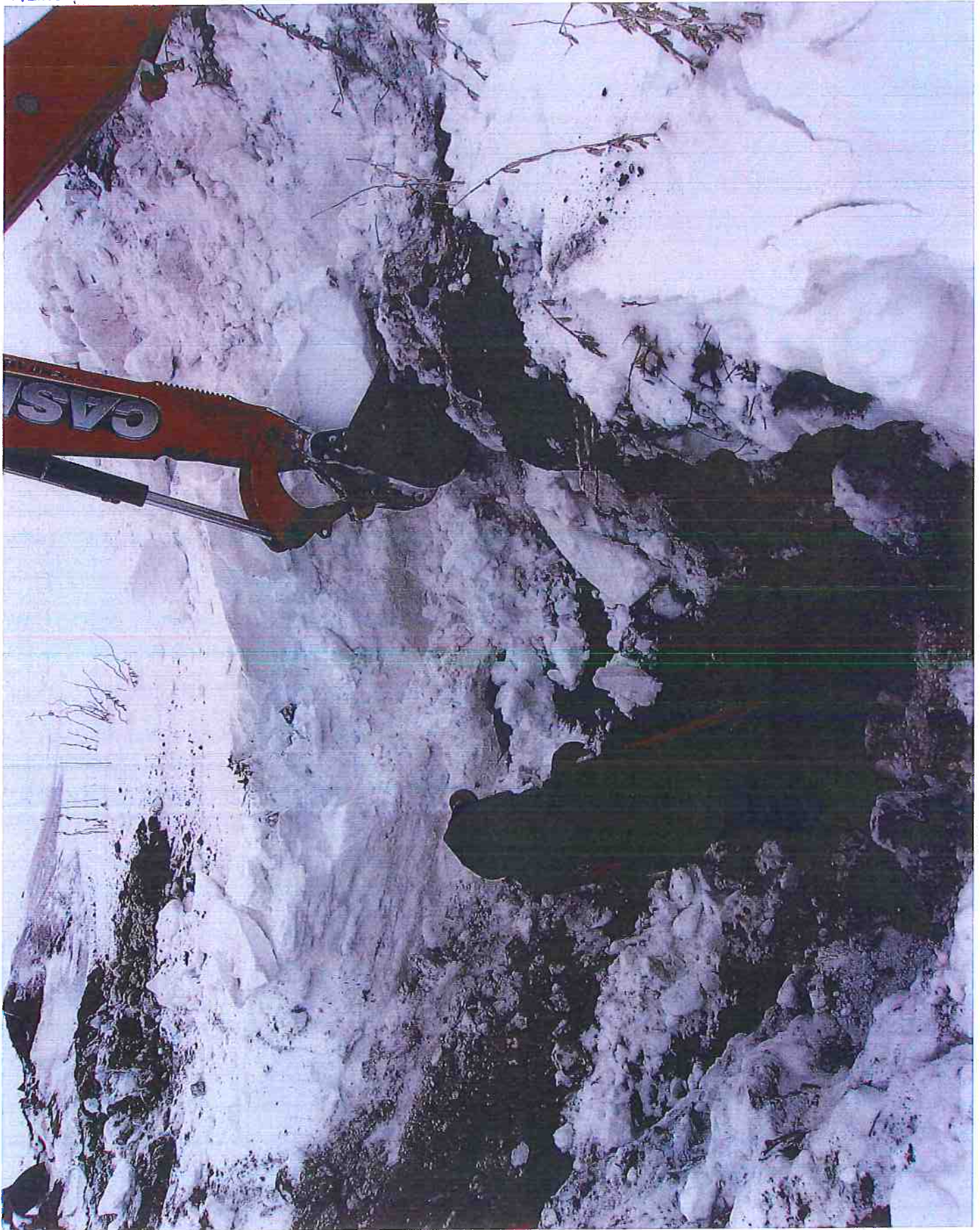
REMOVING SNOW FROM EXISTING HOLE @ #340
