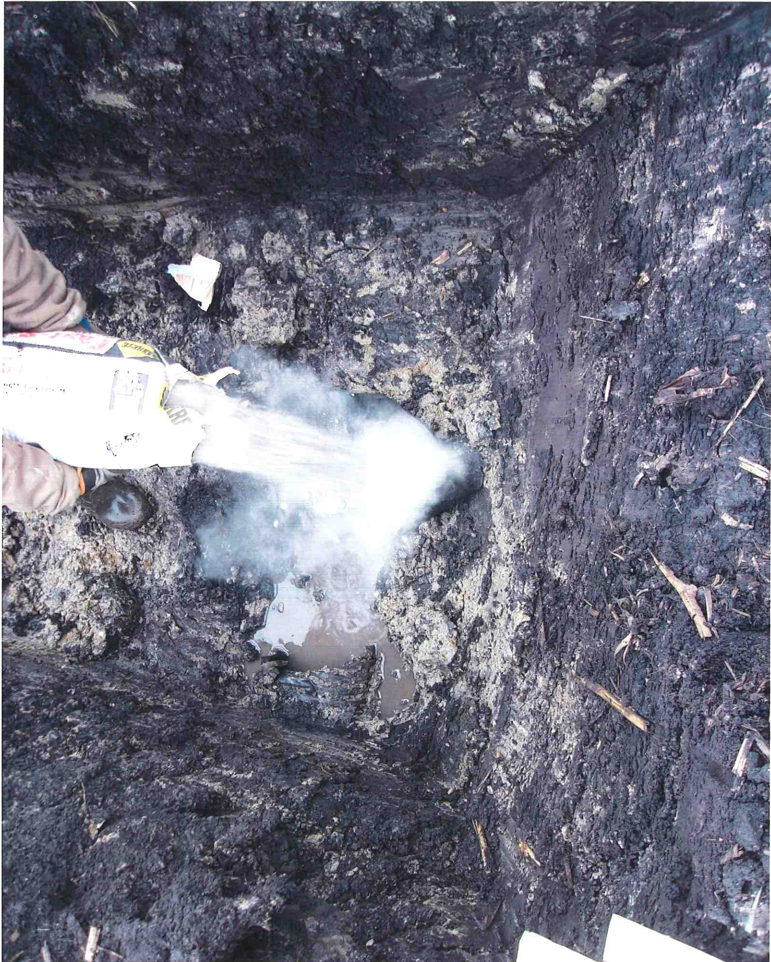
Mix 4 BAGS CONC in Ditch WATER FOR PLOG
